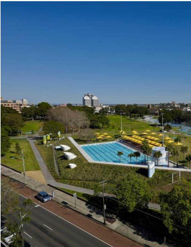
Prince Alfred Park Pool – 2,000m 2 green roof Photo: Brett Boardman
