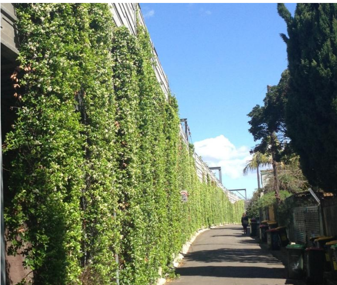
Macdonaldtown rail bridge – green wall
