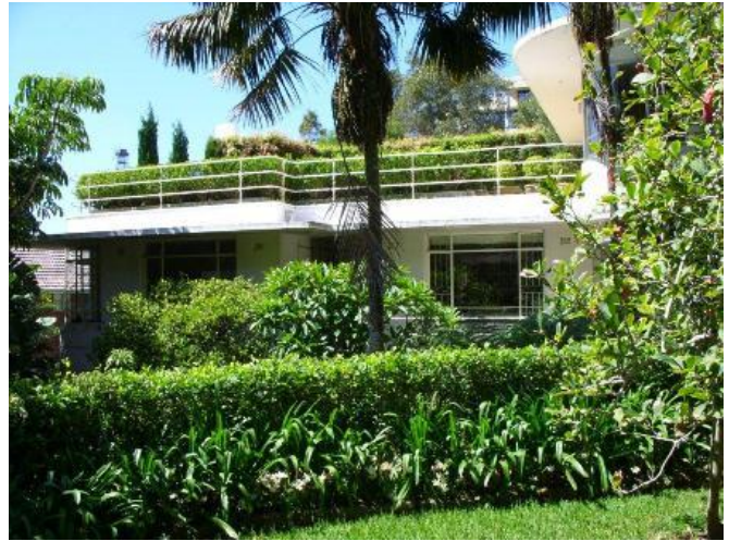
Wyldefel Gardens Potts Point – built 1936 Photo: J Poulton
