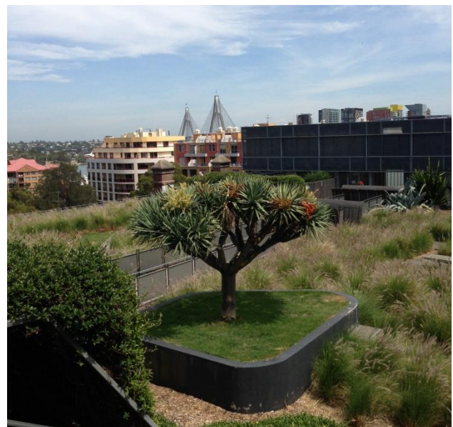
M-Central – Green Roof - Ultimo
